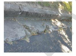
Figure 3-23 Damaged Kerb (Simpson Street)
