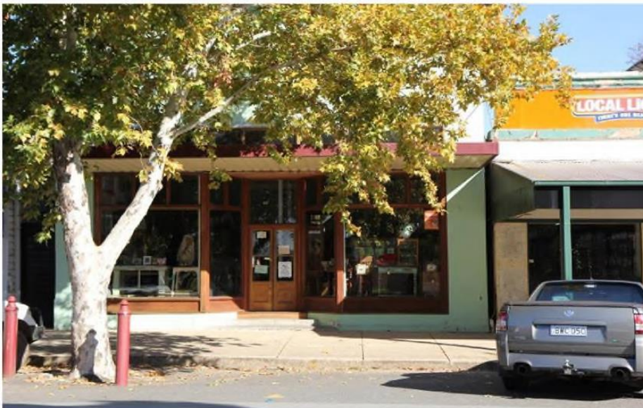
Photograph 19 – Integrating new shop fronts into original building design
