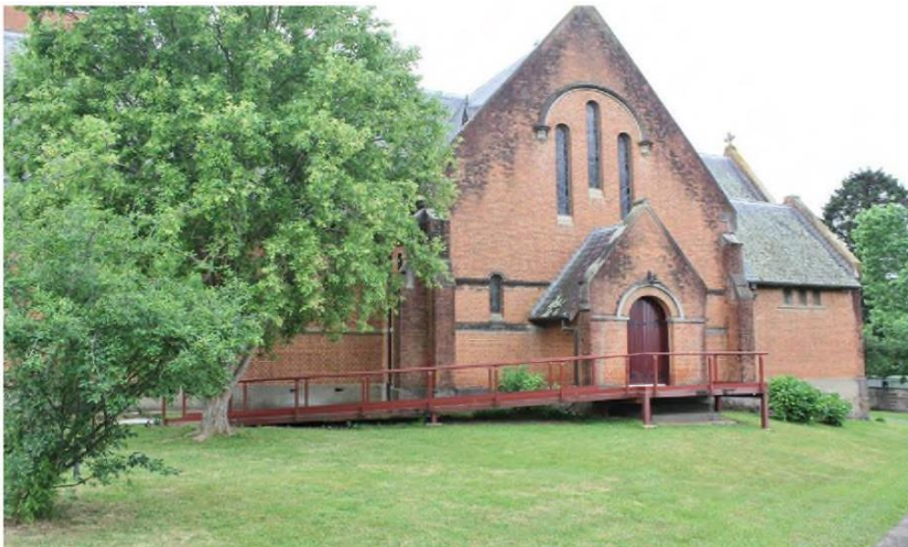
Photograph 18 – Alterations to accommodate access must consider the characteristics of the building
